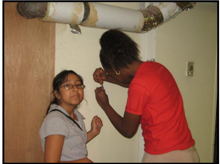
Heather Hernandez and Jasmine Harris repairing the wall
